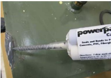
Apply PowerPatch® Sealant over putty patch or leak area
