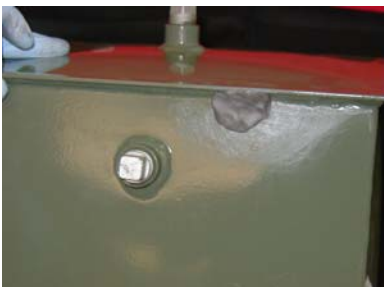
Apply putty 1/2 inch beyond leak; 1/8 to 1/4 inch thick
