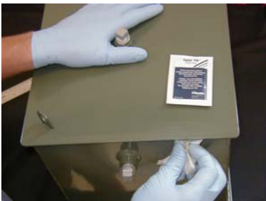
Clean area with Type TR™ before applying PowerPatch ® Putty
